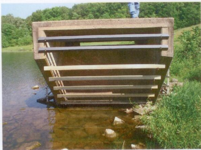
Photograph No. 4: The principal spillway riser.
