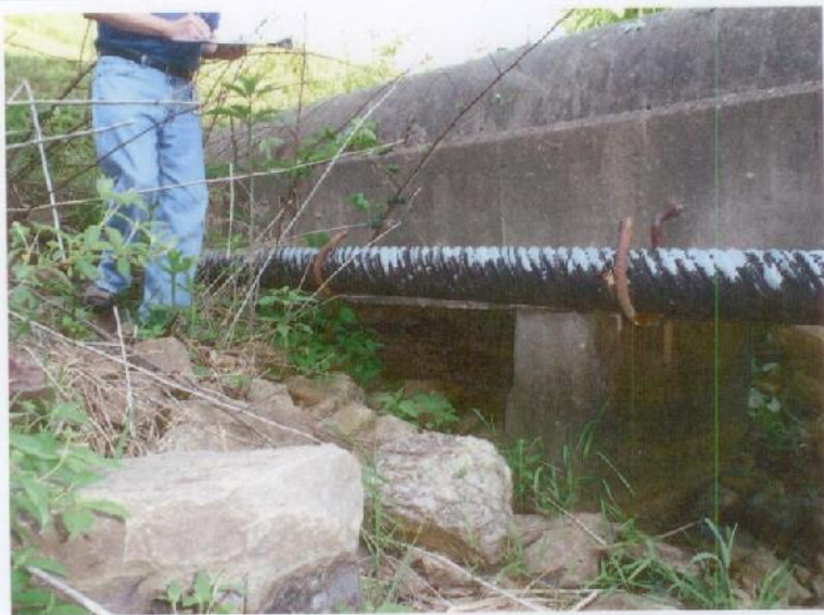
Photograph No. 7: The support for the principal spillway outlet pipe.
