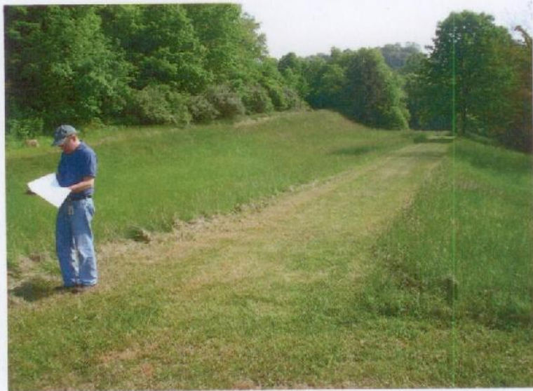
Photograph No. 9: The emergency spillway channel looking downstream.
