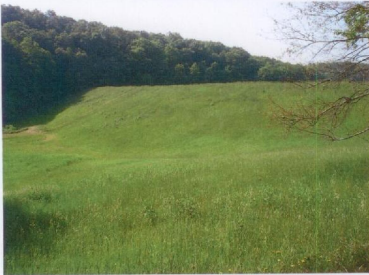
Photograph No. 2: The downstream slope of the dam viewed from the left abutment.
