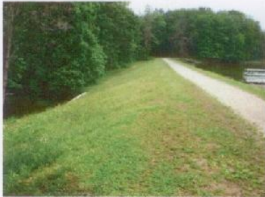
Dam embankment prior to severe flood.
