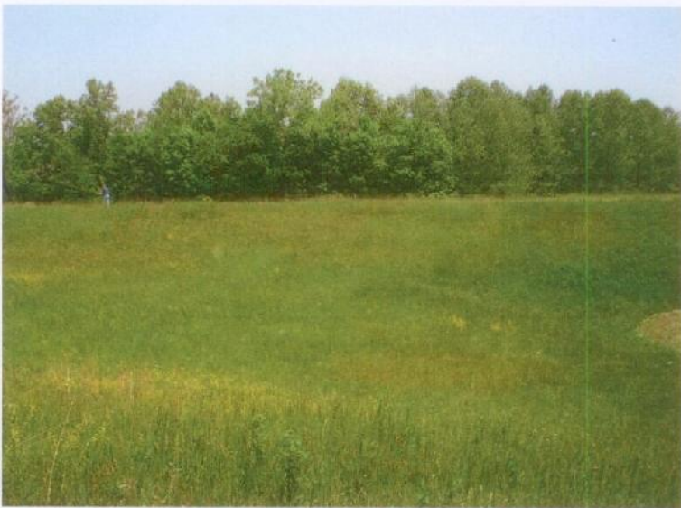
Photograph No. 8: The inlet of the emergency spillway channel.
