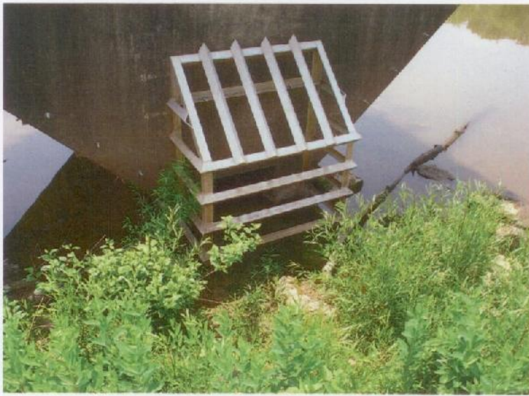
Photograph No. 4: The low-flow inlet of the principal spillway riser.
