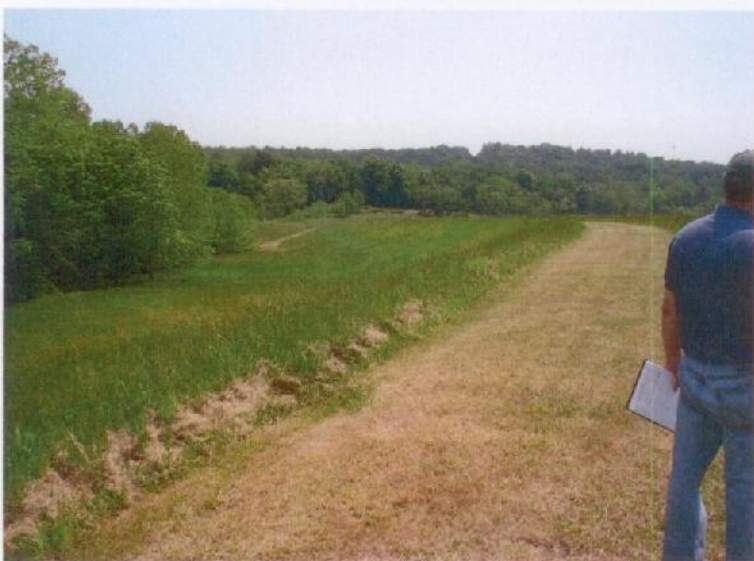
Photograph No. 3: The crest and the downstream slope of the dam.
