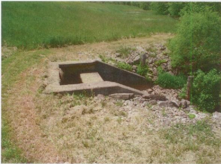
Photograph No. 5: The impact basin at the principal spillway outlet.
