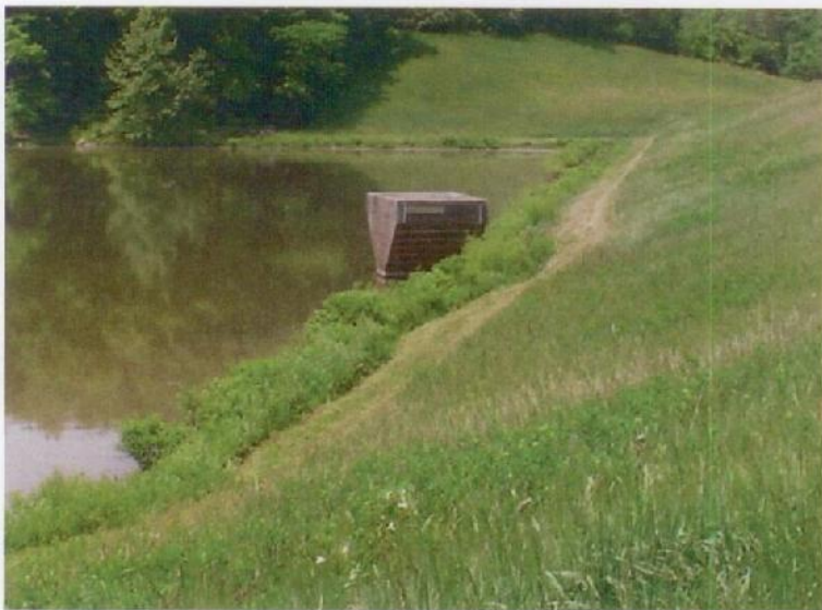
Photograph No. 2: The upstream slope and the principal spillway inlet. Note the brush along the shoreline.
