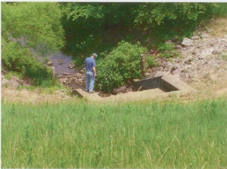
Photograph No. 6: The impact basin at the principal spillway outlet.
