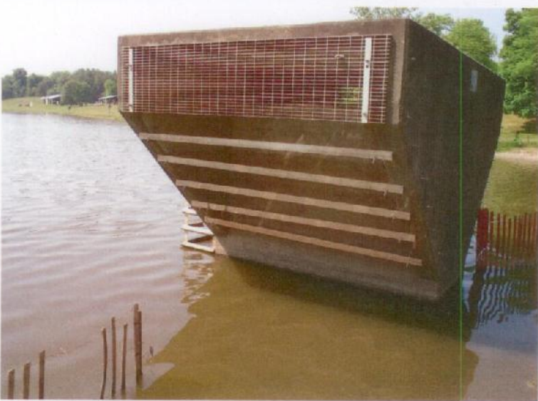
Photograph No. 3: The principal spillway riser.
