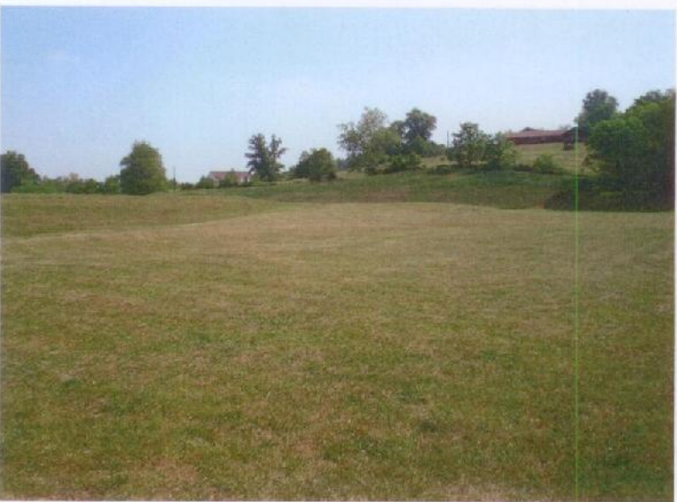
Photograph No. 6: The emergency spillway channel looking downstream.
