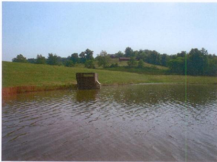
Photograph No. 1: The upstream slope of the dam.
