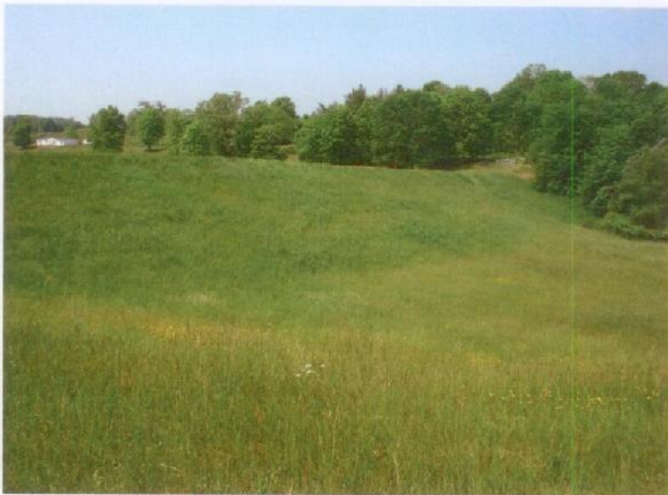
Photograph No. 2: The downstream slope of the dam.
