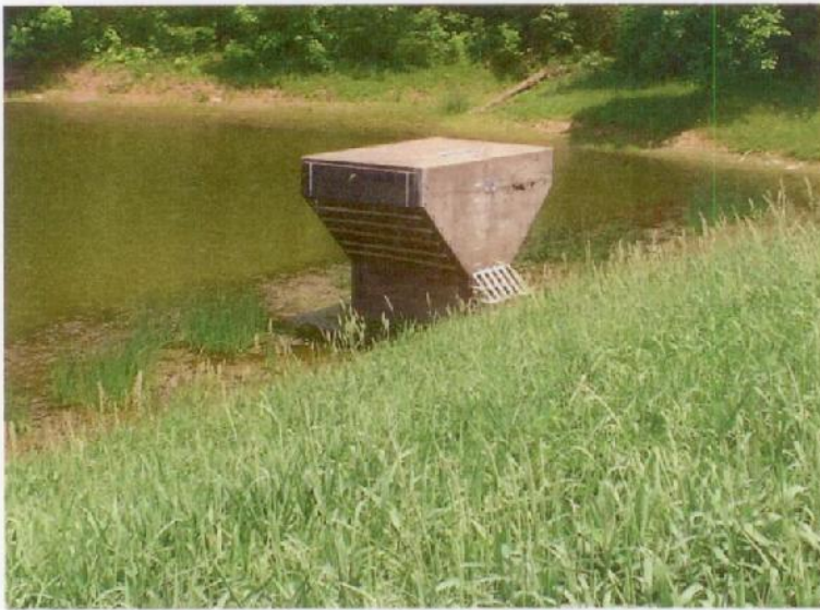
Photograph No. 2: The principal spillway riser.
