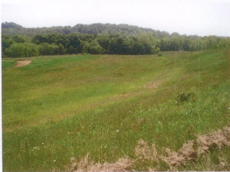
Photograph No. 8: The emergency spillway channel looking downstream.
