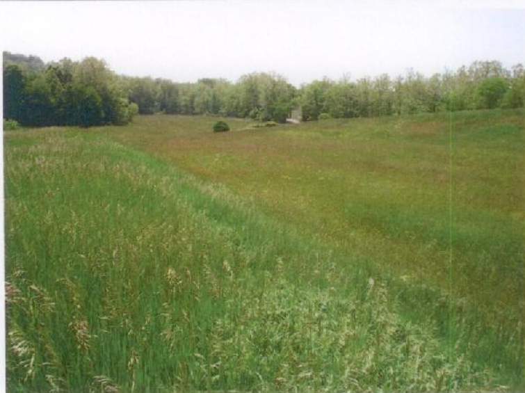
Photograph No. 9: The principal spillway channel looking downstream.
