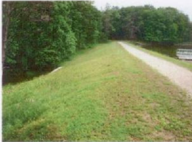
Dam embankment prior to severe flood.
