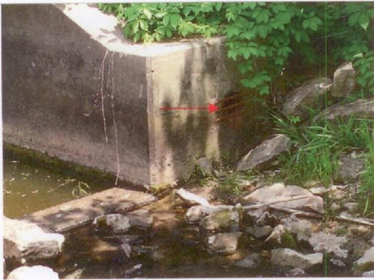
Photograph No. 7: The left toe drain outlet.
