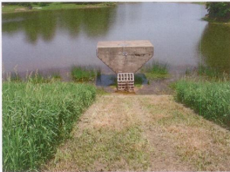
Photograph No. 3: The principal spillway riser.
